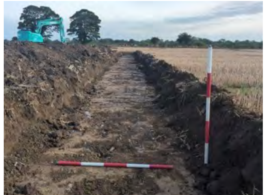
Plate 44: Trench 52, looking south-southwest
