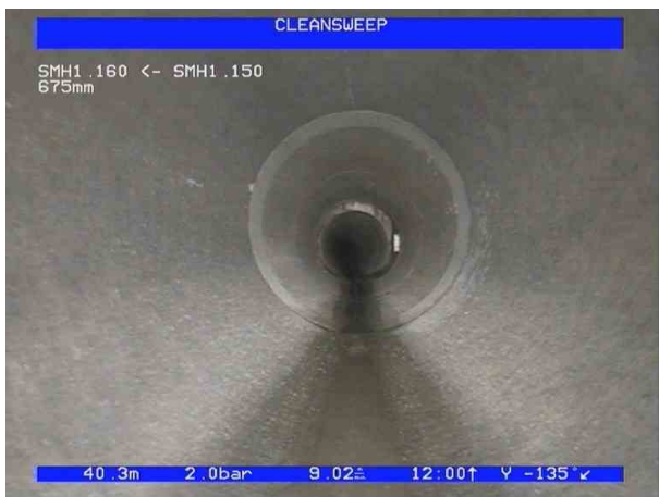
3, 00:04:22, 40.30 m General photograph taken at this point, Condition Photo
