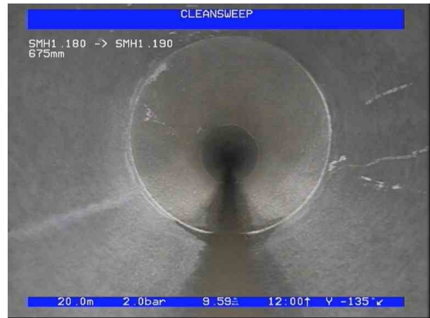
2, 00:02:01, 20.00 m General photograph taken at this point, Condition Photo
