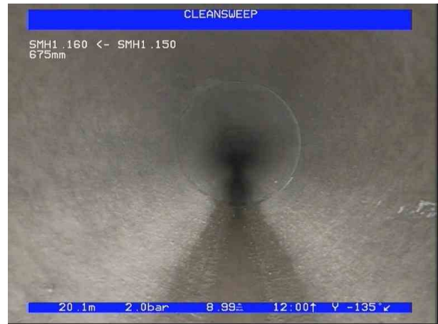
2, 00:02:10, 20.10 m General photograph taken at this point, Condition Photo
