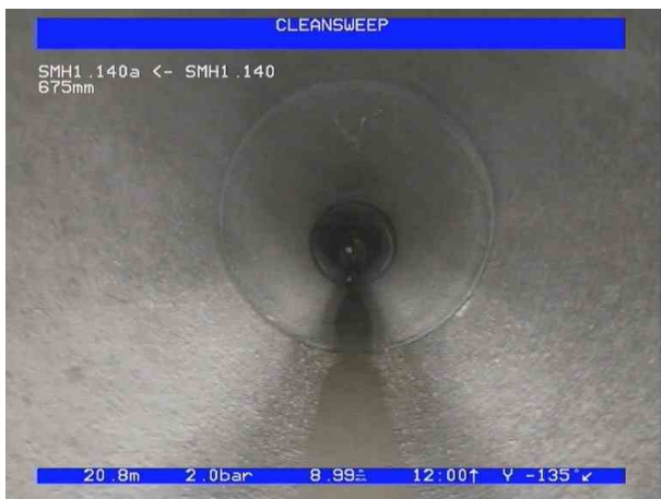
3, 00:02:26, 20.80 m General photograph taken at this point, Condition Photo
