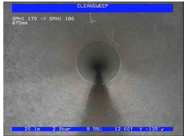
2, 00:02:12, 20.10 m General photograph taken at this point, Condition Photo
