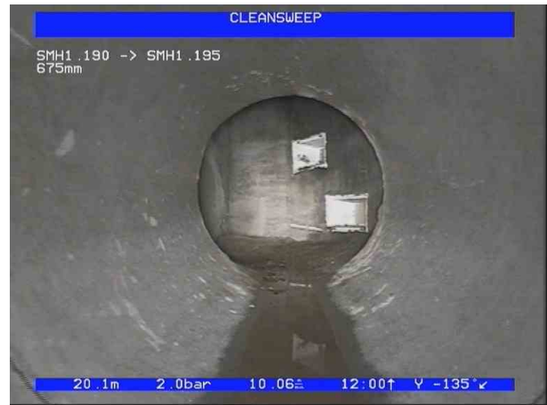
2, 00:01:57, 20.10 m General photograph taken at this point, Condition Photo
