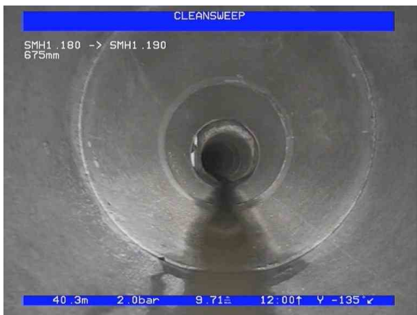
3, 00:04:08, 40.30 m General photograph taken at this point, Condition Photo
