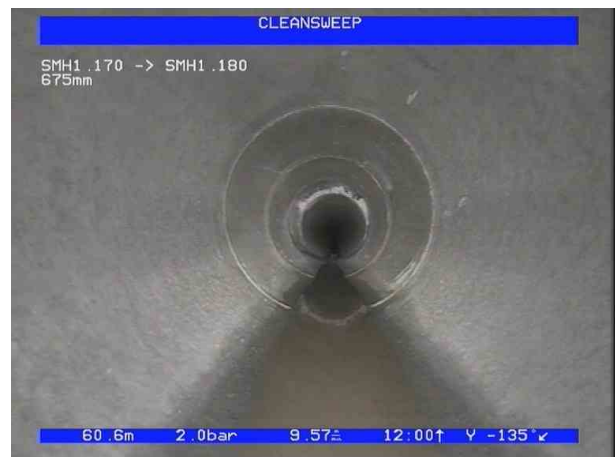
4, 00:06:17, 60.60 m General photograph taken at this point, Condition Photo
