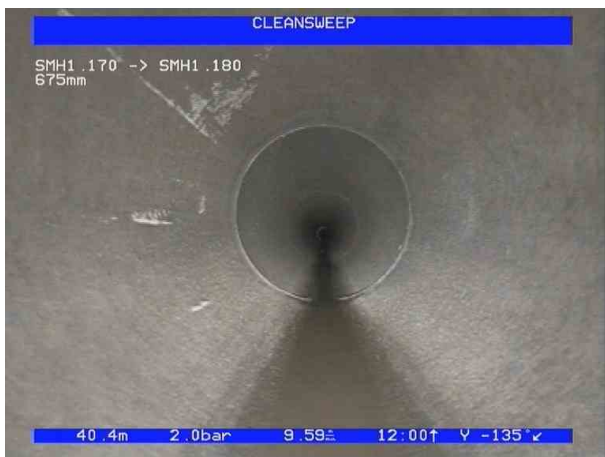
3, 00:04:15, 40.40 m General photograph taken at this point, Condition Photo
