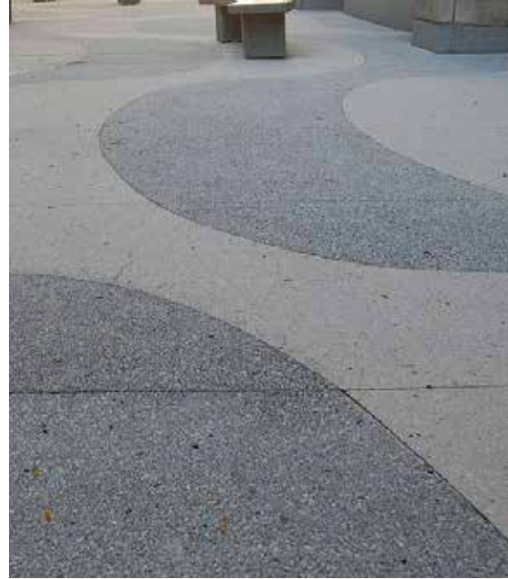
2 In situ exposed concrete
