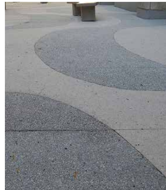
6 2 tone concrete paving
