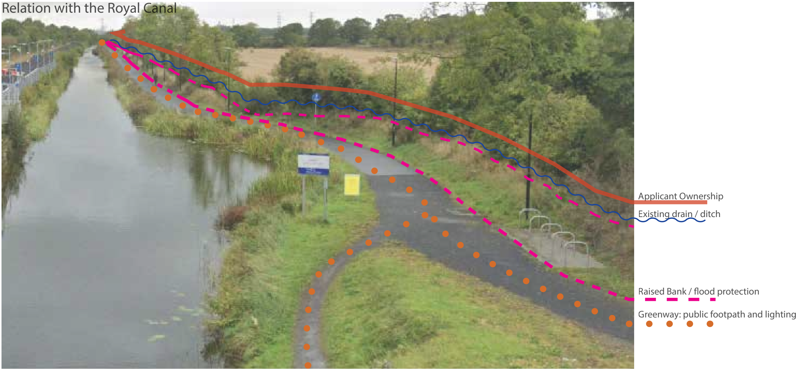
Street view from the bridge looking West
