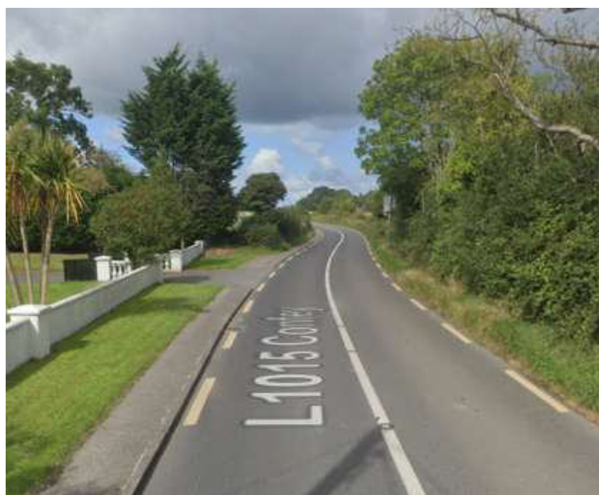
Figure 4 –L1015 Confey Road (no existing public lighting)
