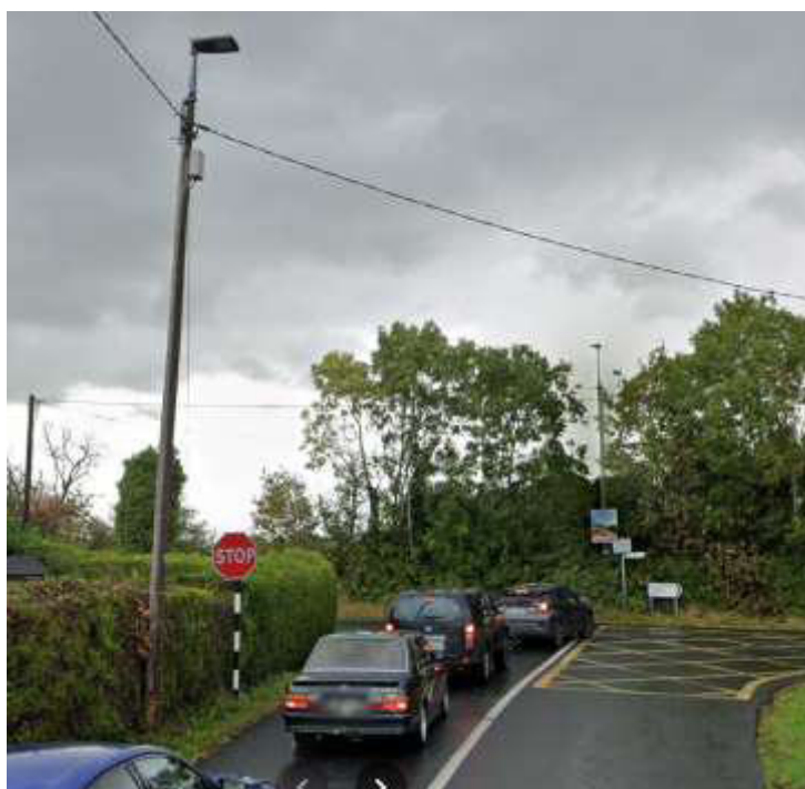
Figure 3 – R149 / L1015 Roads Junction Existing LED Lighting (to be retained)
